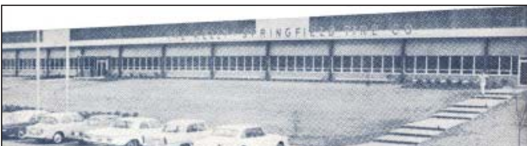
The front of the plant looks much like it does today. Of course the Kelly Springfield sign is gone and the cars parked in front today are a little more modern than the ones in the picture.
