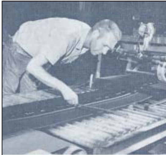
TUBER OPERATOR shown in this photo is checking tread width to set up a production run
